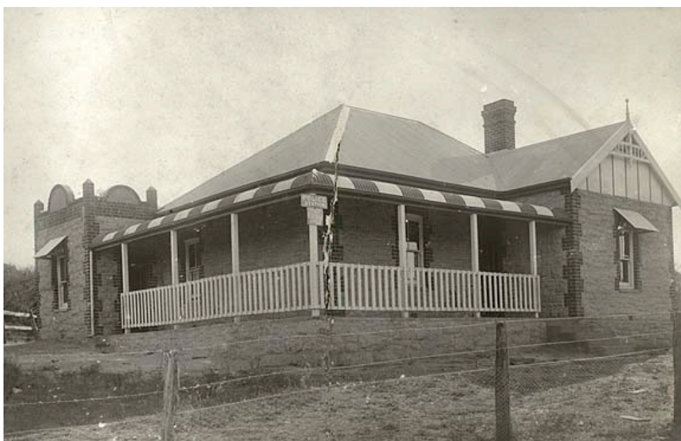
Rugby Police Station, NSW – No date
